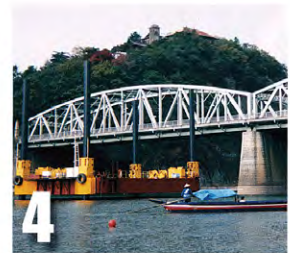
4 Completion (construction of lower portion of New Inuyama Bridge)
