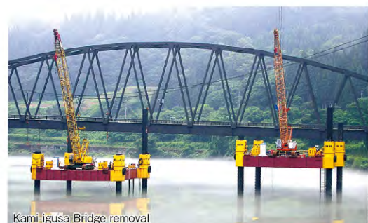
Kami-igusa Bridge removal
