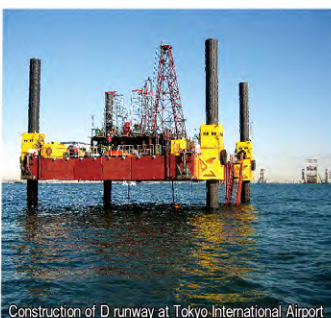
Construction of D runway at Tokyo International Airport
