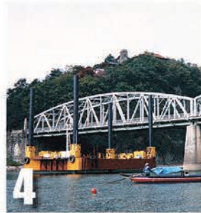
4 [完成(新犬山橋下部工事)]
